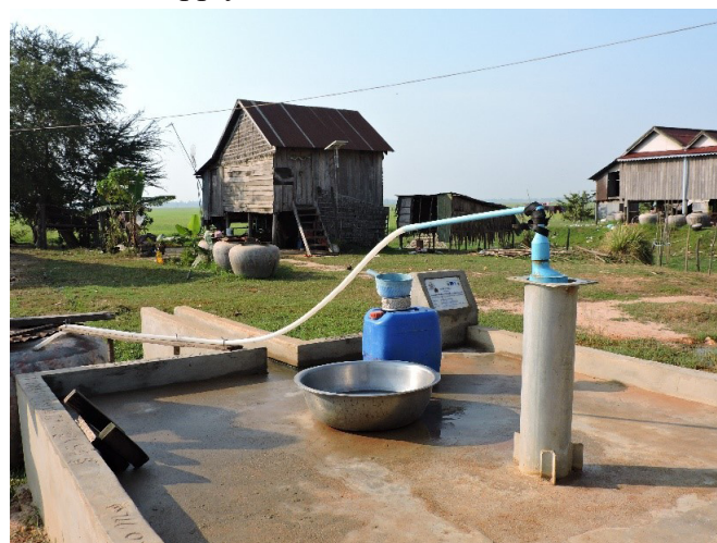
Figure 2: Deep drilled well for year-round water supply
