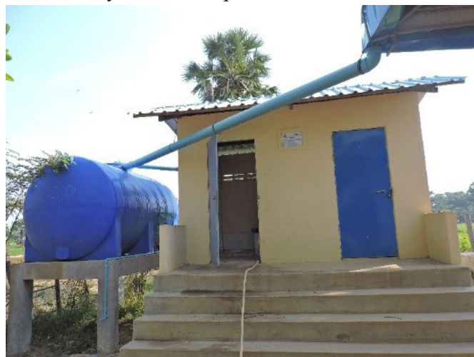
Figure 3: Latrine and rainwater collection/storage system for improved sanitation
