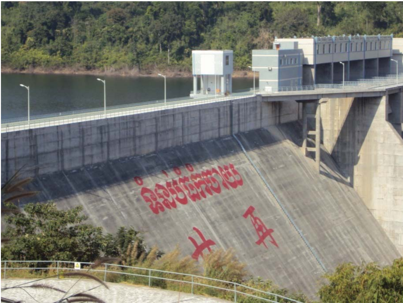
Figure 1: Kamchay hydropower dam, Kampot province
